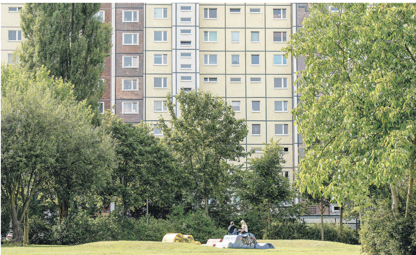
Betonburg in Hellersdorf Foto: Maurizio Gambarini / picture alliance
